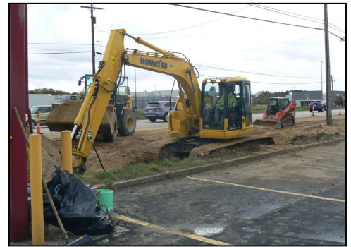
Top: Construction of the water and sewer lines.
