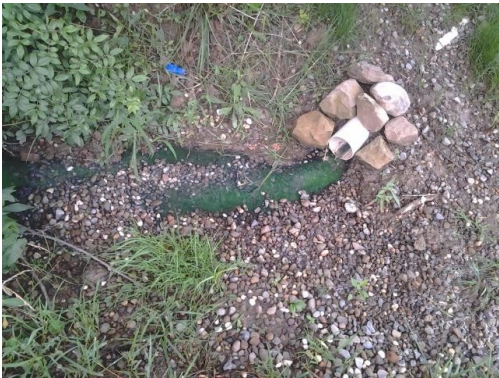
Right: Illicit discharge from common drain pipe taking sewage from neighborhood and dumping waste water onto private property.
