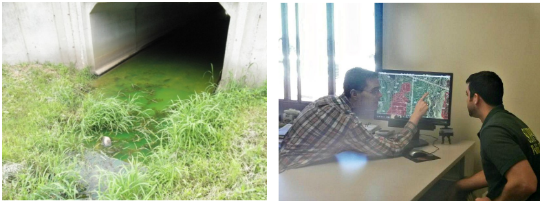
Above: Illicit discharge of wastewater transported from a common ditch tile.
