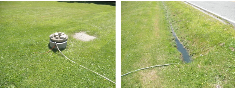
Left: Illicit discharging of wastewater from a septic tank into a roadside ditch.
