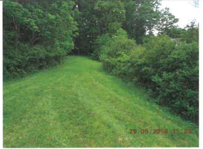
View of the dam crest from the left abutment. Note the dense trees and brush on upstream and downstream slopes.
