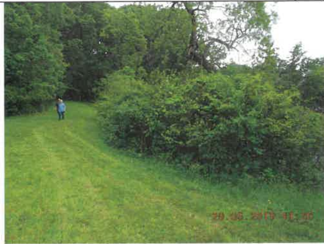
Trees and brush along the upstream slope.
