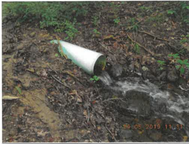
Another view of the principal spillway outlet.
