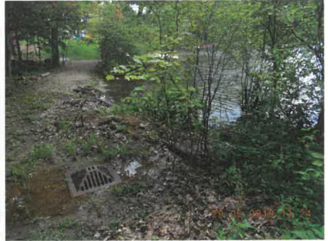
View of the emergency spillway. Note the trees and brush at the inlet.
