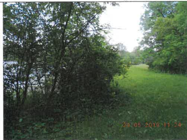
View of the upstream slope and crest from the right abutment. Again notice the trees and brush on the slopes.
