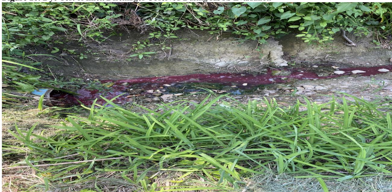
Figure 16: Dye Test of Illicit Discharges Observed During HSTS Evaluation
